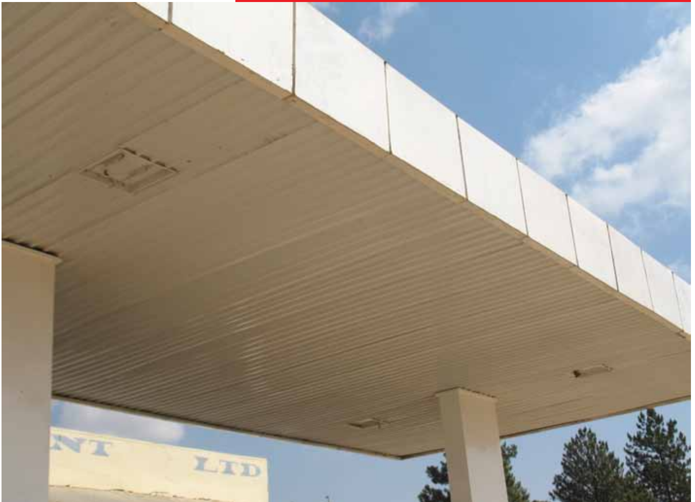
Newly installed canopy at Mount Meru Nakonde filling station
