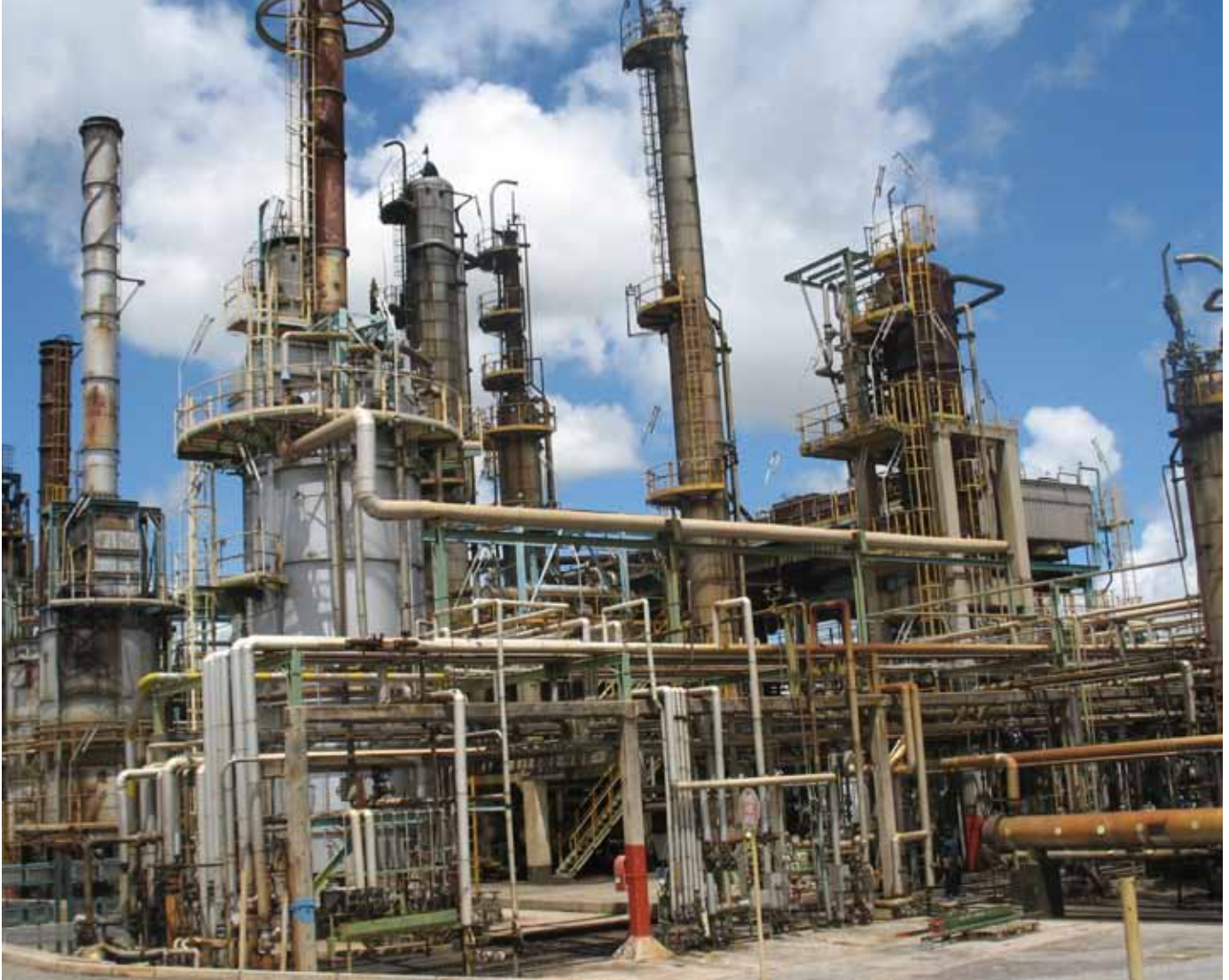
Indeni Oil Refinery in Ndola
